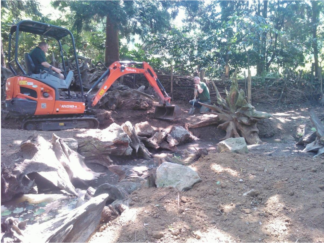
Photograph 4: Construction - creating a soil mound
